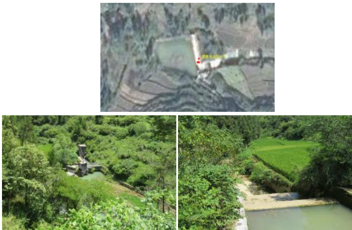
图2.1-9 菱角电站现状
